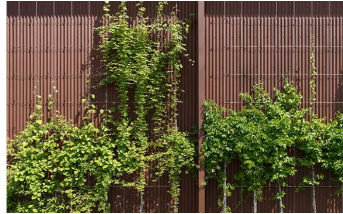
Green screen with steel cable trellis and climbing plant
