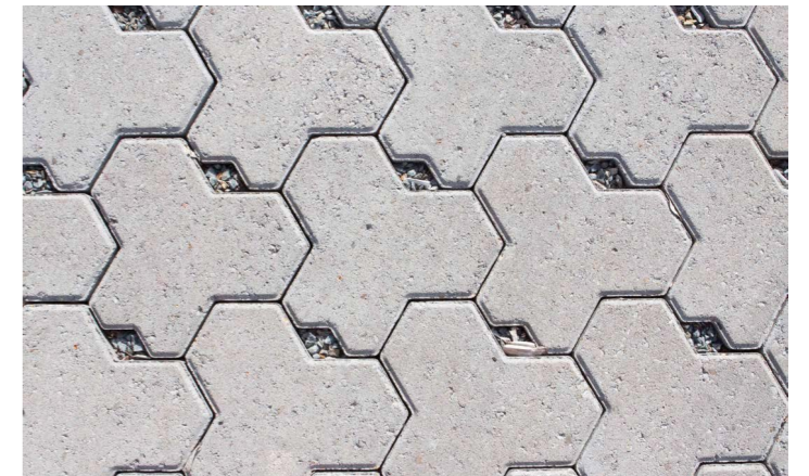
Permeable paving
